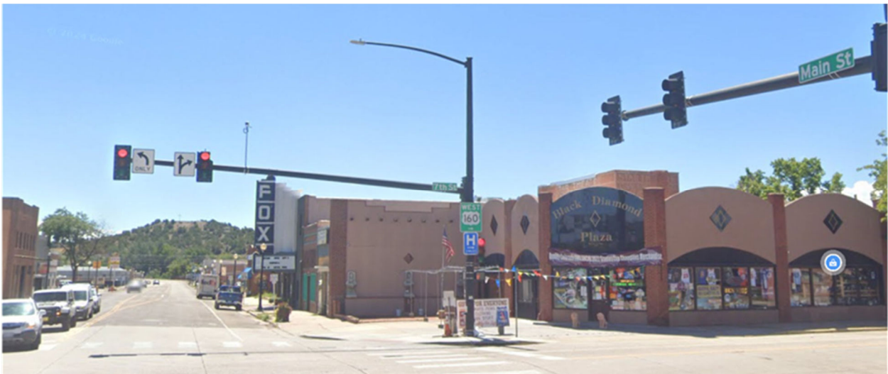
Figure 3-12. Signal Head Condition
